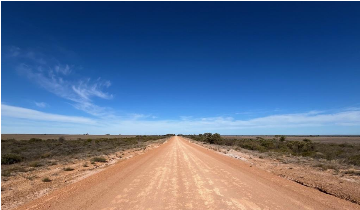
Figure 9: looking south along Mt Adams Road, with carriageway in centre of R10876 and 40-metre wide kwongan vegetation on either side. IDHS 26/5/26
