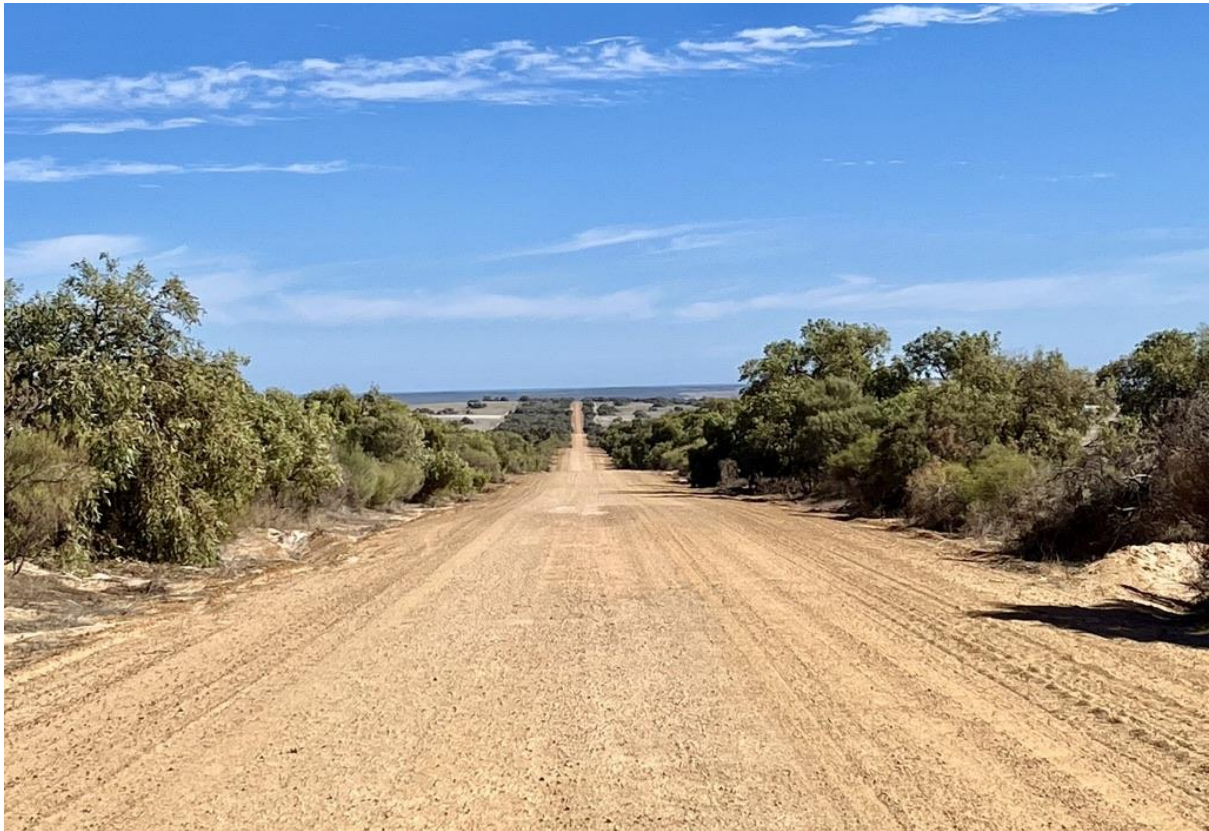
Figure 7: Yandanooka Road looking west from Mt Adams, showing same widths of R10876 and carriageway as looking east, with remnant Pricklybark woodland. IDHS 26/5/26
